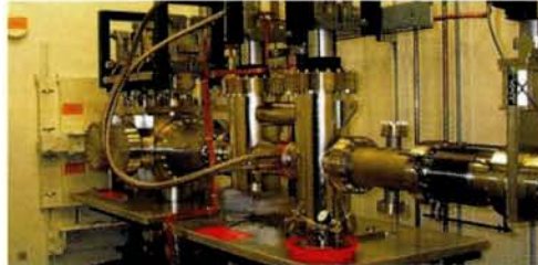
Beam line components for Advanced Photon Source
