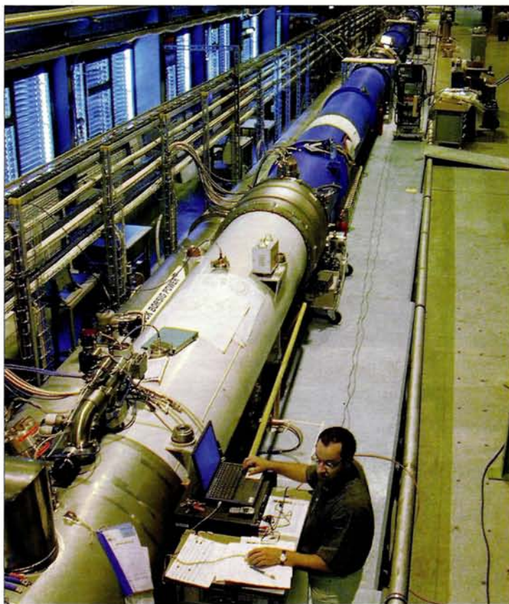
The String 2 test installation for CERN's Large Hadron Collider.
